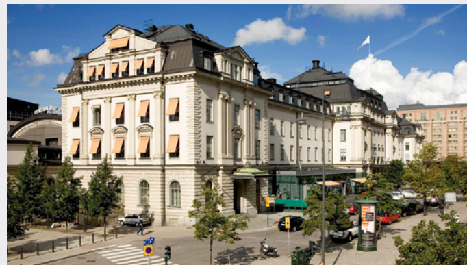
Jernhusen manages all its building information over a lifecycle perspective using Service Works Global's FM system. Image: Stockholm Central Station, a Jernhusen property.
